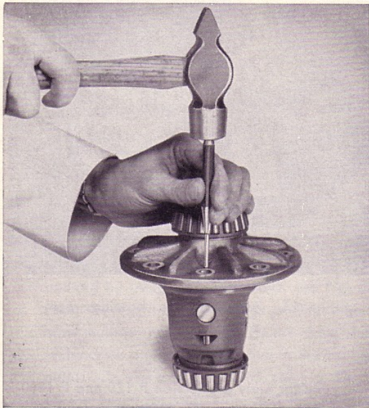
Fig. 15. Removing the locking pin.
